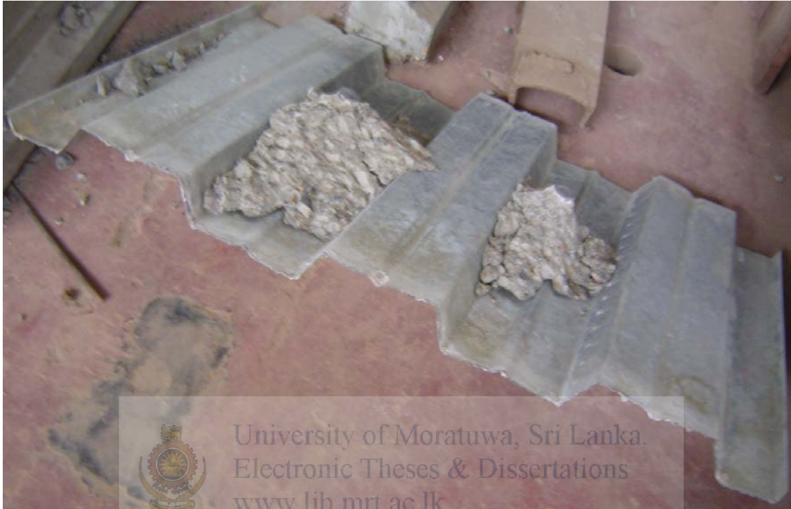
Figure 4.19: Wedge Cone and Pyramid Cone Failure
