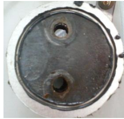
Figure 9 – Corroded Al plate after a test run for 24 h with 30 g of KOH applied (500 ml water)
