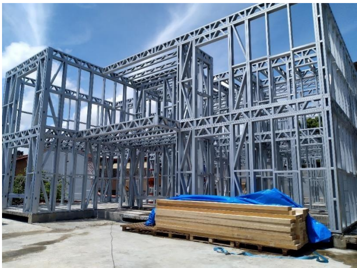
Figure 2: Wall frames in a cold formed steel building
