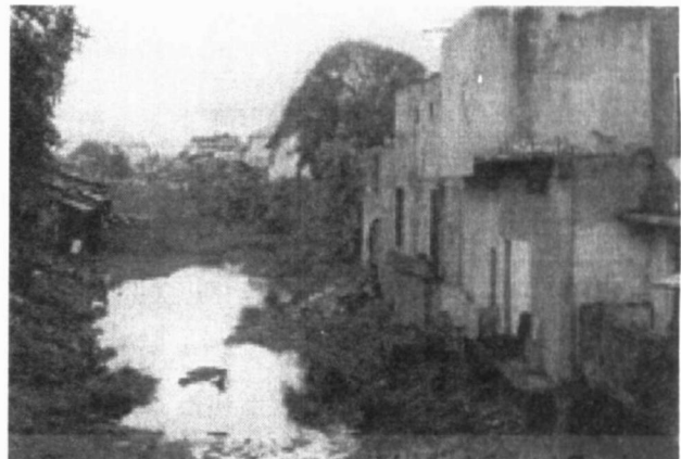
Figure 2: Previous Condition of Canal Banks (photo credits: Herath, 1996)
