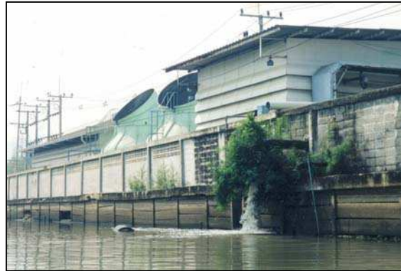
Figure 5: Industrial effluent discharge to canal
