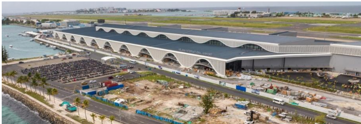
Fig. 4. Maldives International Airport, new terminal building, North-East Birds eye view, Image from Digital Twin
