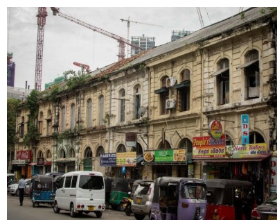
Fig. 2,3 Demolished state of the De Zoysa Building
