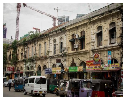
Fig. 2,3 Demolished state of the De Zoysa Building
