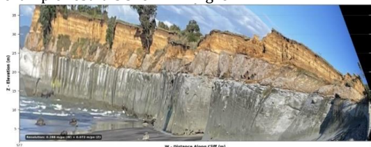
Figure 6. Example geo-rectified cliff image for the Ōnaero site, obtained by projecting the smartphone photograph onto the fitted cubic-polynomial cliff surface and registering the output to the NZTM coordinate system.
